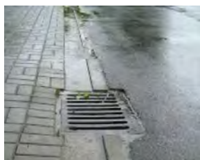
Photo: Example of a typical catch basin inlet
